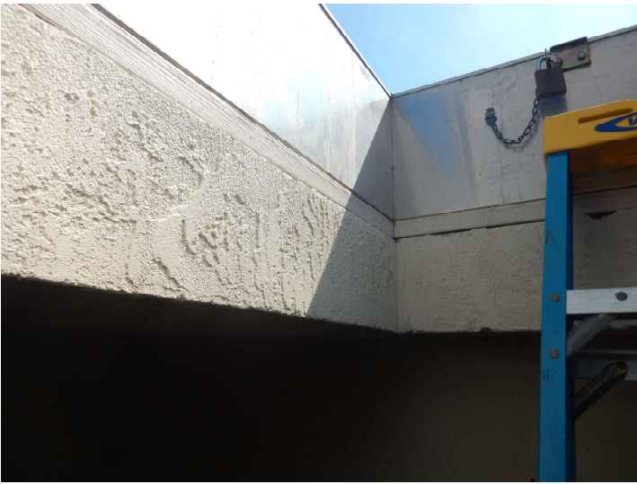
Concrete Roof Deck
