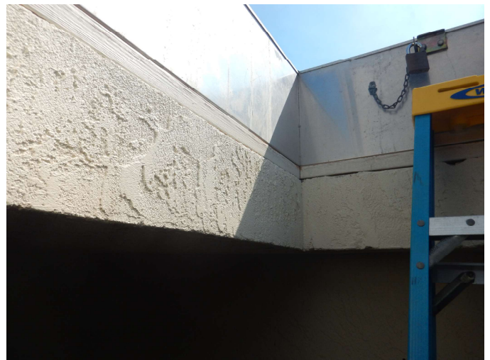
Concrete Roof Deck
