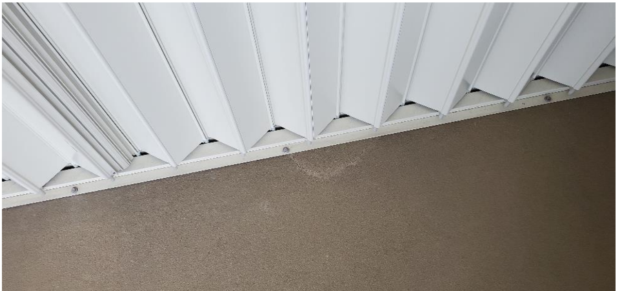
Concrete spall under shutter track caused by reinforcing steel corrosion
