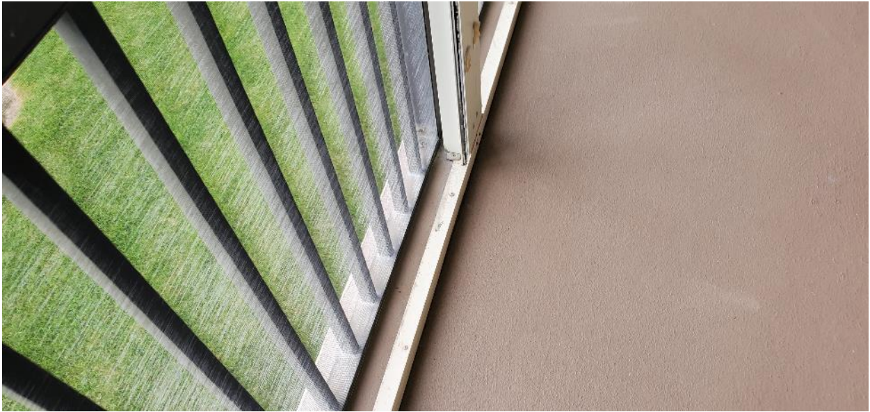
Shutters at balcony edge properly shimmed
